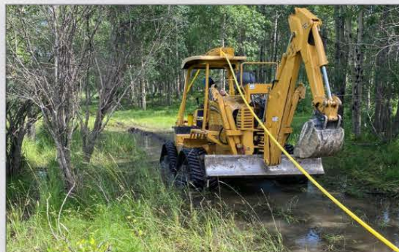
Vibratory plow gas line installation
