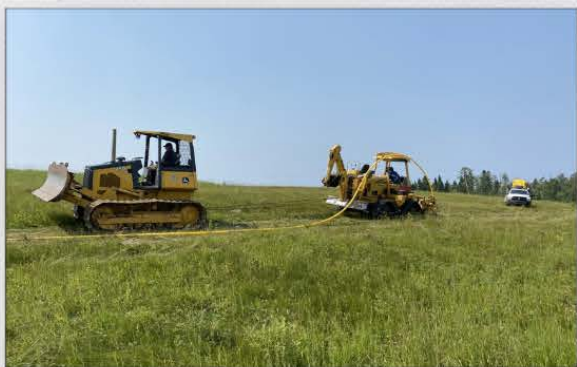
The construction team at work
