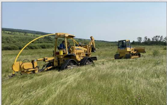
Loop line being installed
